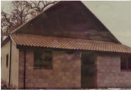
Building the new village hall.
