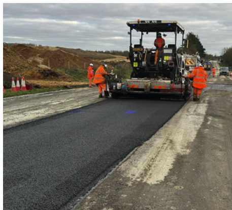
Work on the A47. Picture: National Highways
